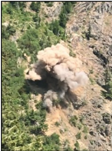
Dust cloud from explosive detonation to improve tread Photo by Kyle Hannah
