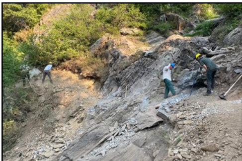
Trail Crew working on Leigh Lake Trail
